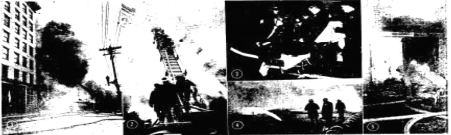
Here are scenes from the most fatal fire in Charleston's history, which occurred Tuesday night in front of the Woolworth building on Canal St. as flames and streams of water poured from the sky to bring the structure down.
