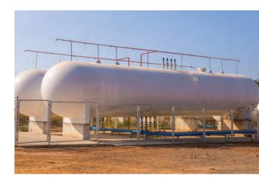
odorant added. An odorant is added when LPG is offloaded to a distribution system or transport tanks to permit detection of vapor leakage.
