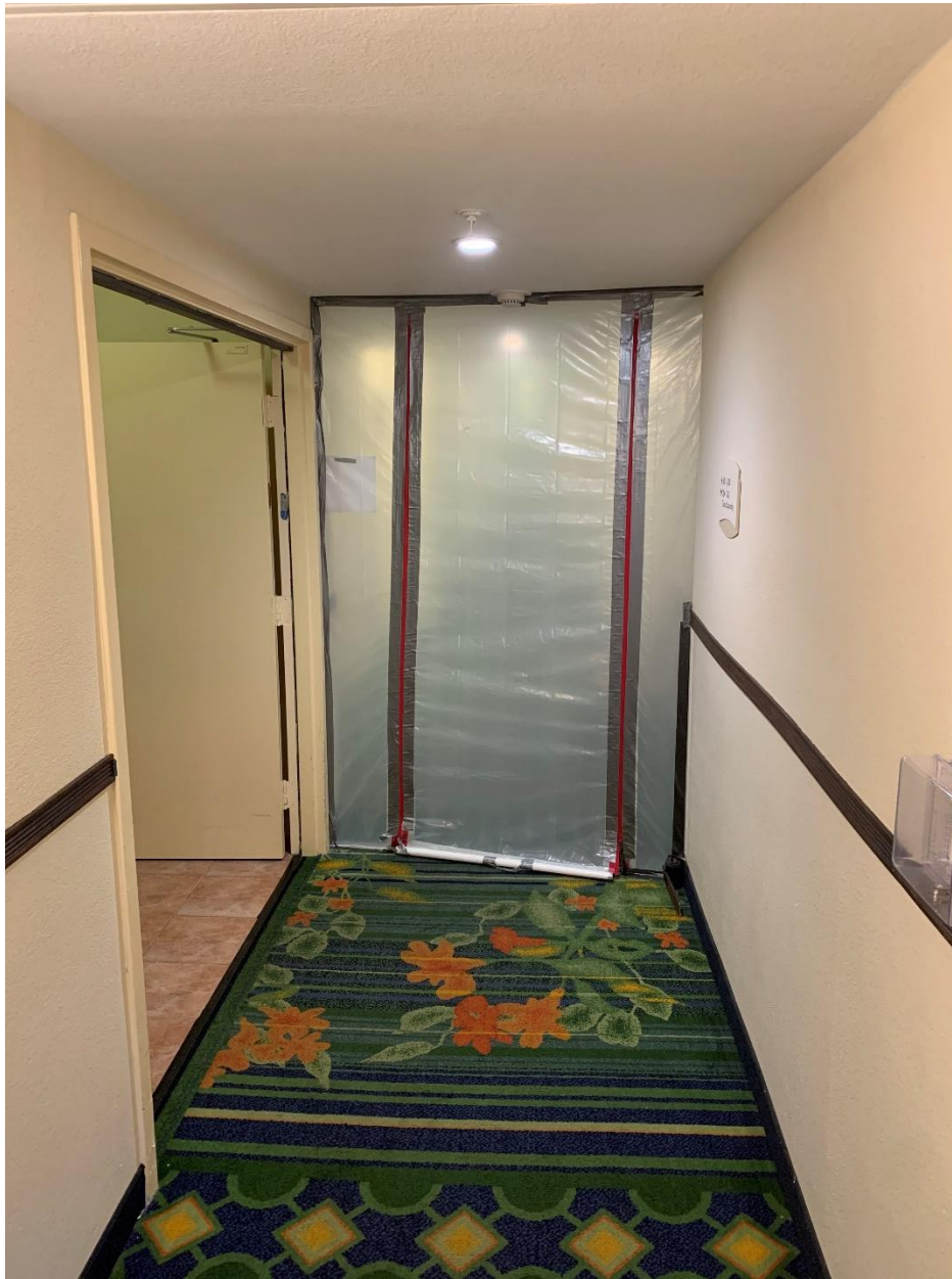
Figure 3: Sample Plastic Barrier to Isolation Zone Area
