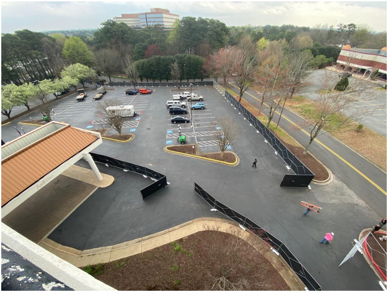
Figure 1: Site Perimeter Fencing
