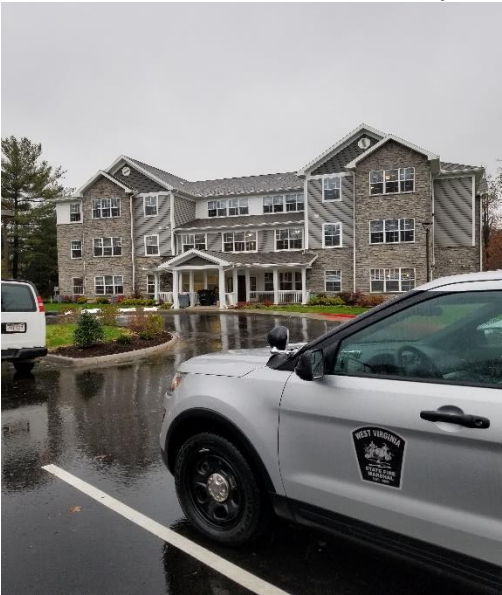
Newberry Apartments – Wood County
