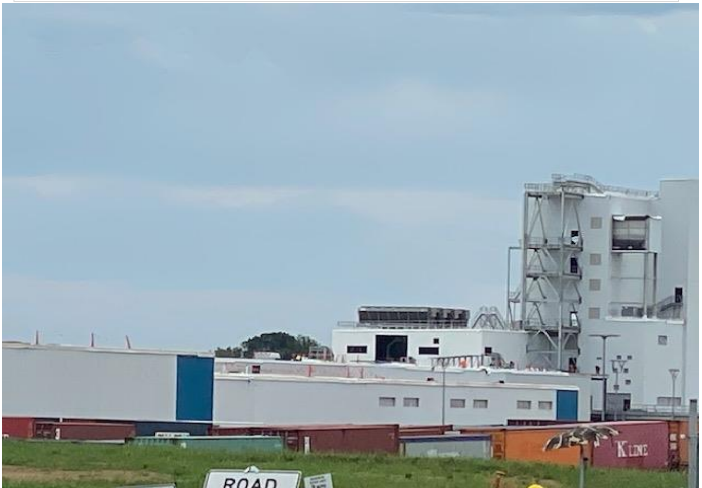
Rockwool Insulation Manufacturing Company - Ranson
