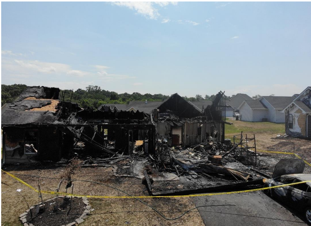
Berkeley County/Photo by ASFM Harms
