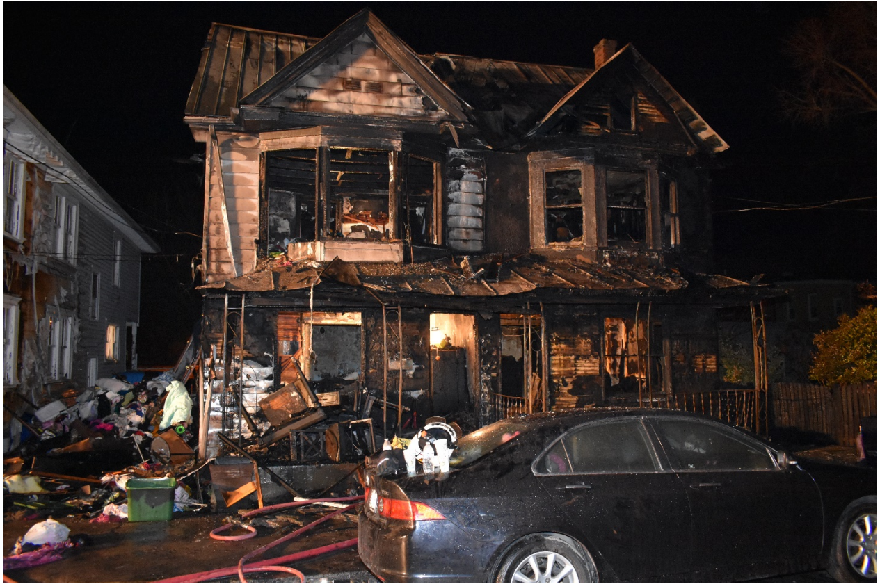
Berkeley County/Photo by ASFM Harms
