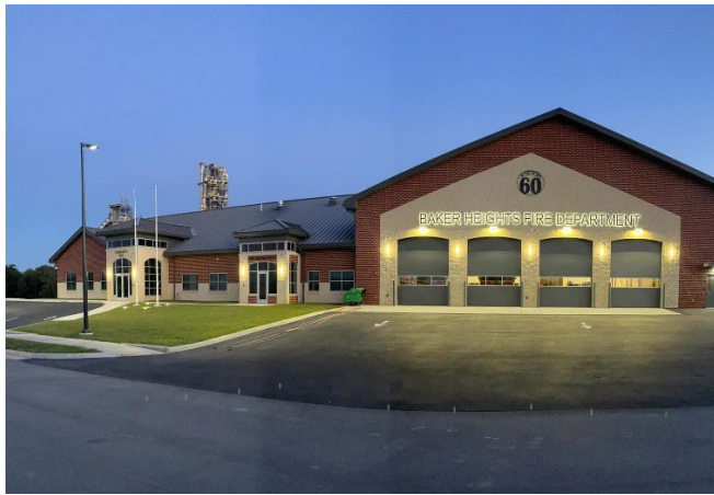
Baker Heights VFD – Berkeley County
