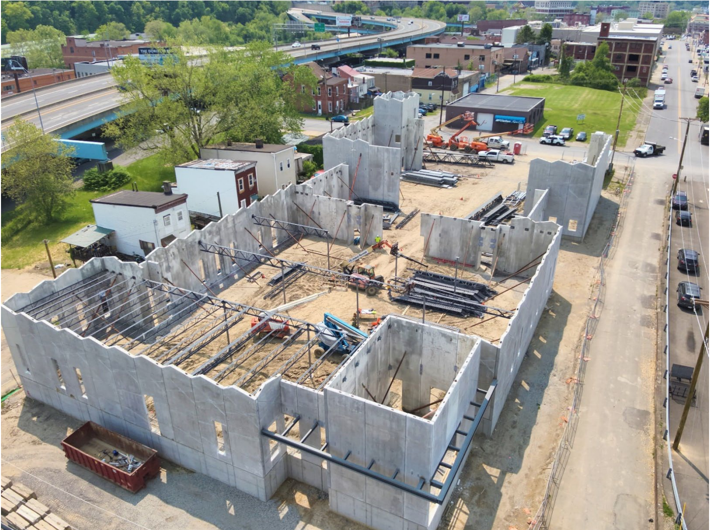
Aerial view of the new Wheeling Fire Department Headquarters
